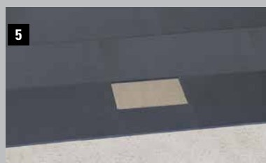
Fit the lining
