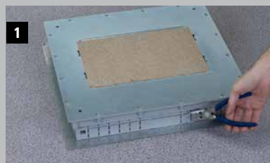
Trim the trunking entries
